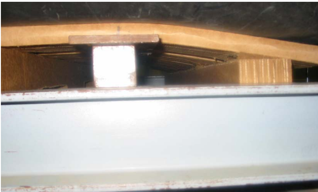
Figure 5: Failure of the Pallet Engineering pallet occurring outside the edge of the fork tine when tested to failure.
